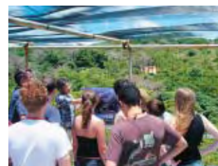
Participants visited the main campus construction site in Onna Village and received a brief orientation from an OIST staff member about the construction plan.
